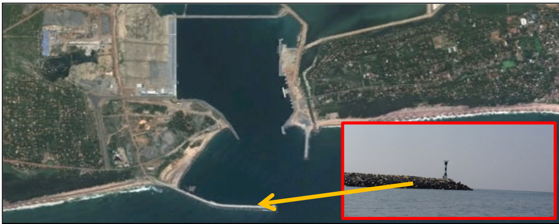
Figure 2.25 Breakwater concrete structures
