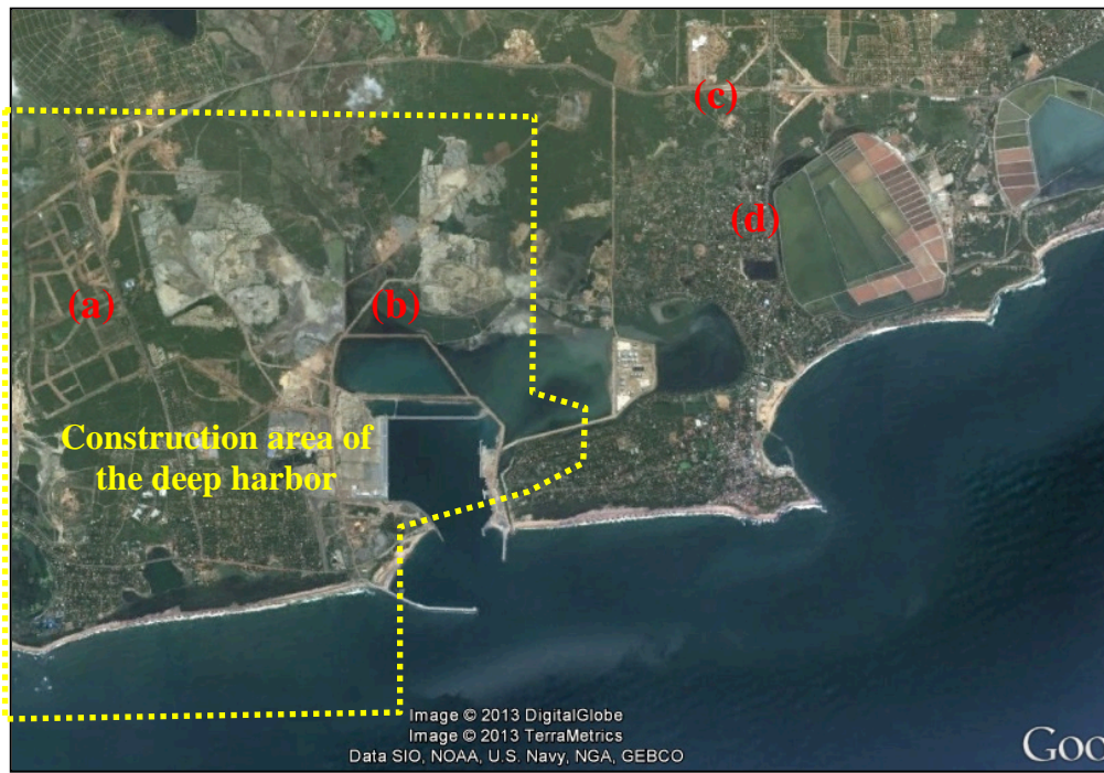
Figure 3.14 Construction area of the deep harbor
