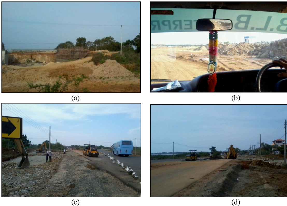
Figure 3.15 Construction sites in Hambantota
