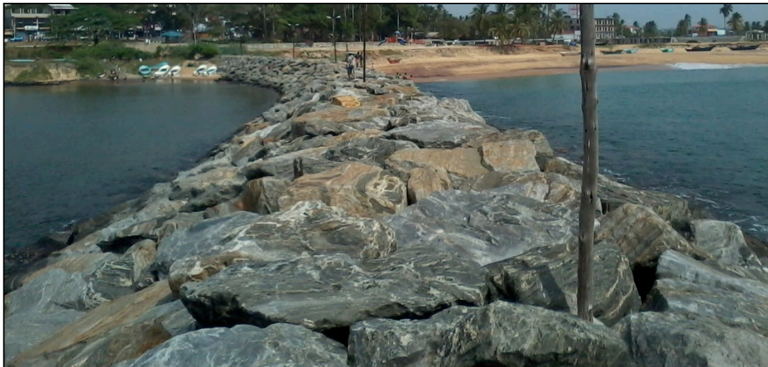
Figure 4.4 surveyor on the breakwater structure/barrier
