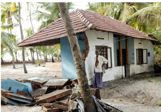
Figure 6.11 Damage Level 2 (Severe damage) for non-solid building
