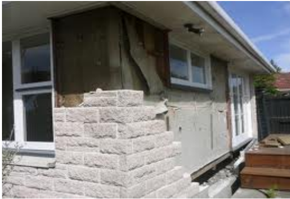
Figure 6.9 Damage Level 0 (No damage to superficial damage) for non-solid building
