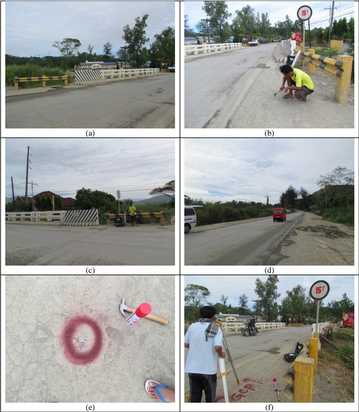
Figure 3.7 GPS static survey condition above GCP1
