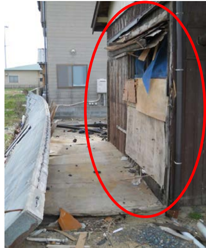
Figure 6.9 Damage Level 0 (No damage to superficial damage) for non-solid building
