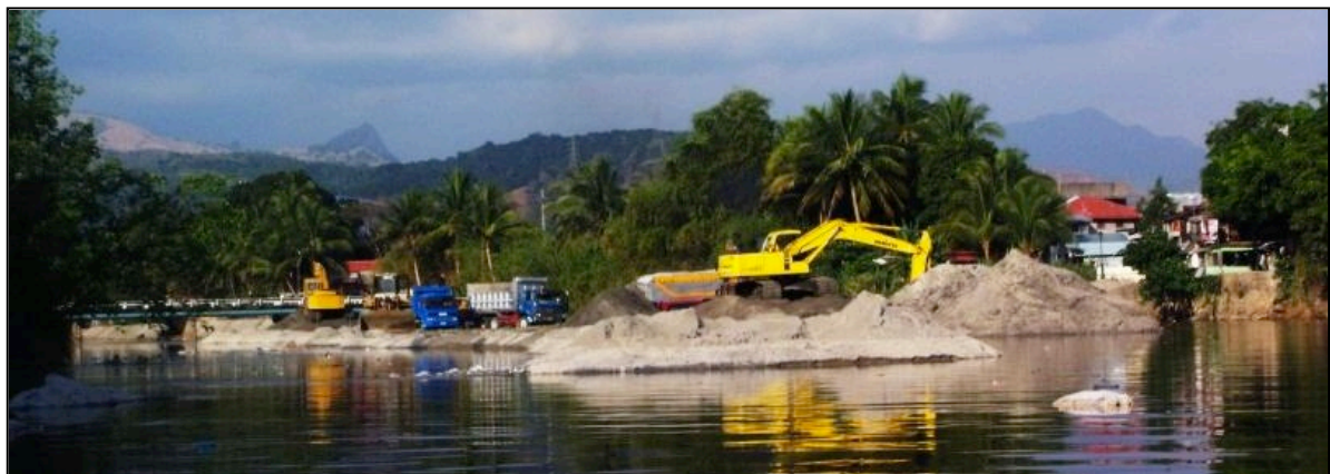
Figure 5.5 Dredging of lahar deposits
