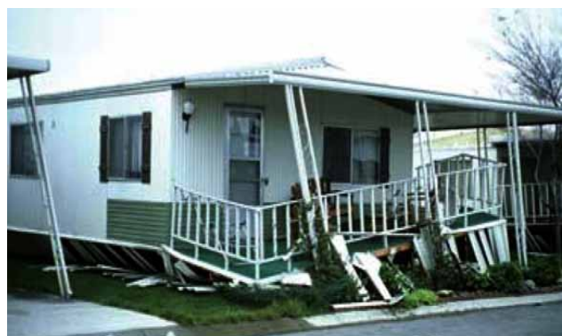
Figure 6.11 Damage Level 2 (Severe damage) for non-solid building
