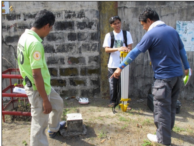
Figure 3.3 GPS setup on a known horizontal benchmark (ZBS-3200)
