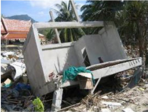
(a) Joint failure
