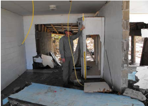
Figure 6.10 Damage Level 1 (Moderate damage) for non-solid building
