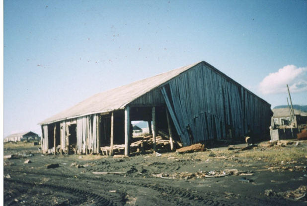
Figure 6.10 Damage Level 1 (Moderate damage) for non-solid building
