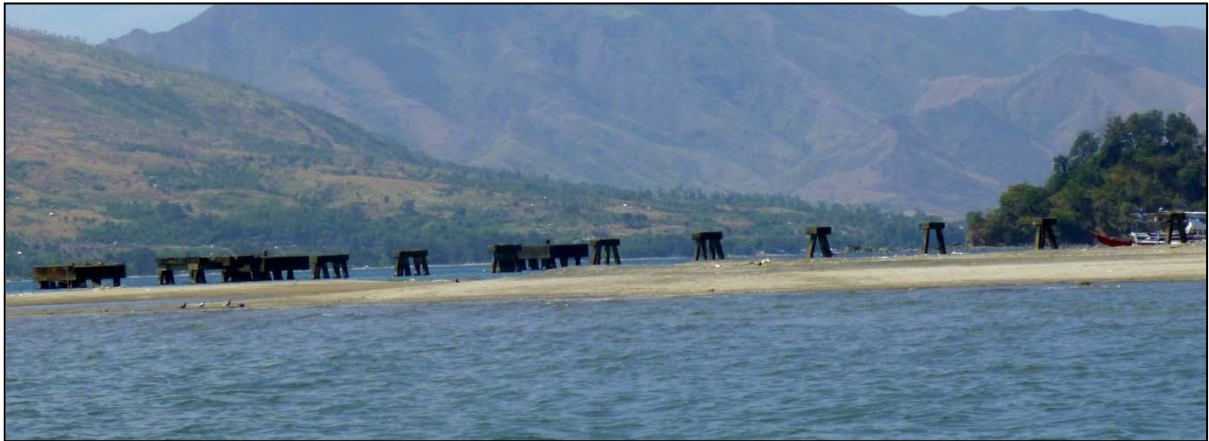
Figure 2.44 Unfinished concrete structure
