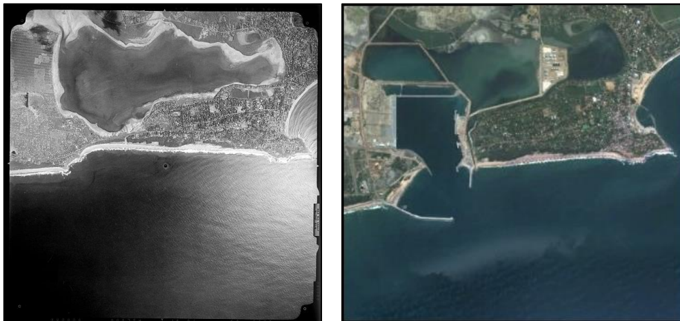
Figure 12. Recent harbor constructions
