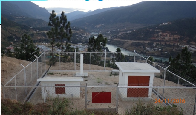
Constructed Seismic stations for Broadband Seismometers, SMA and GNSS receivers
